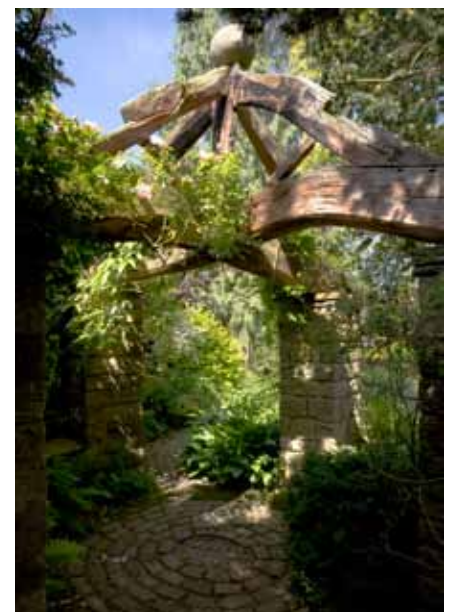
Charred wooden trusses of The Arbour (Photo: John Whitaker)
