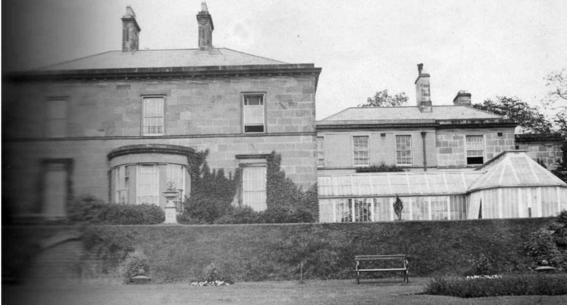
Figure 5 – Cleveland Lodge south front and part of terrace garden undated but before 1901. Source: Frenchay Museum Archives
