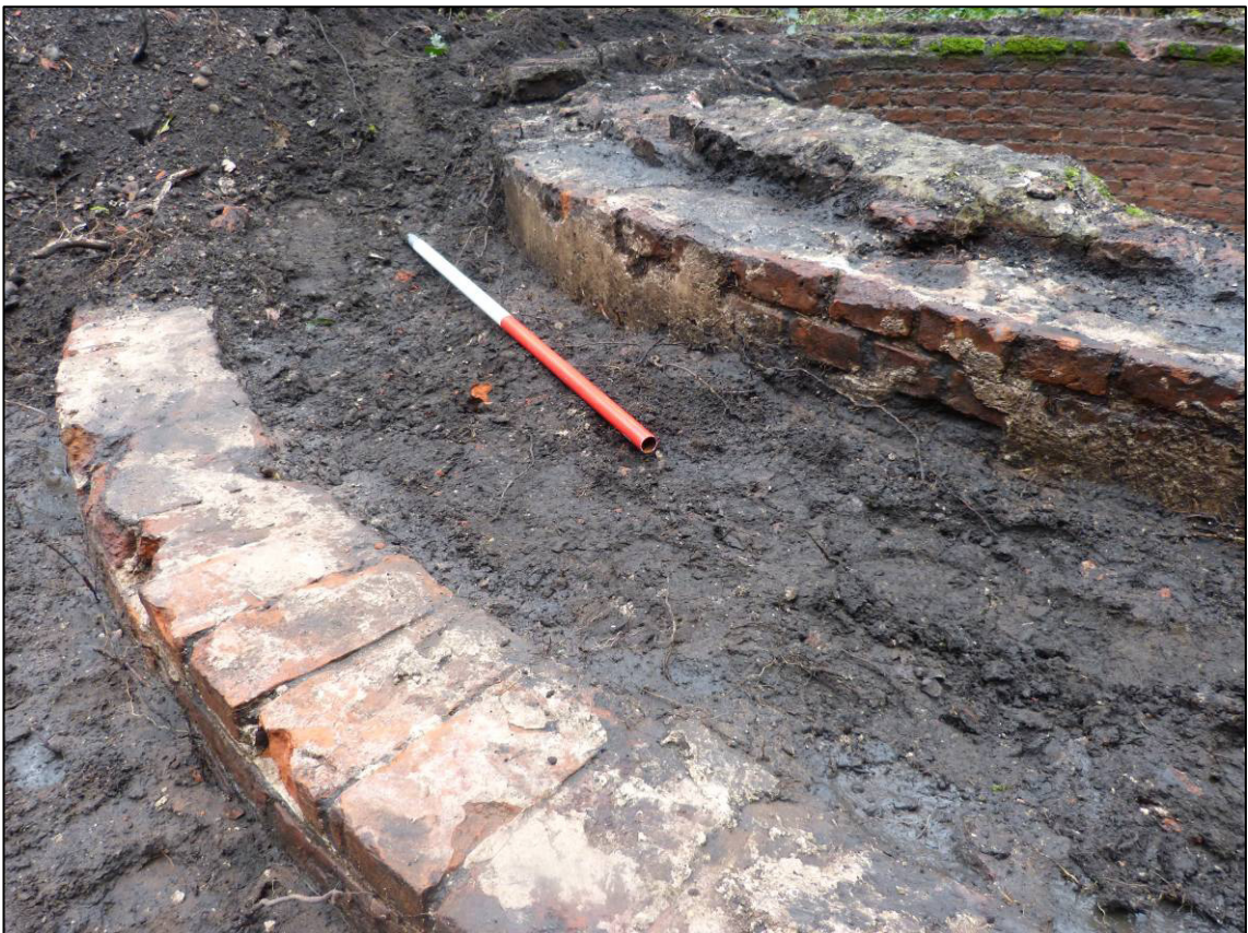
Plate 2: Outer ring of brickwork and render to external face of ice well, looking N (1m scale) (photo 2/216).
