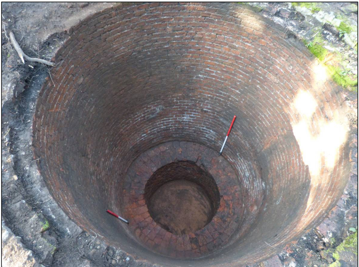
Plate 4: Fully excavated ice well, looking NE (2 x 1m scale) (photo 3/252).
