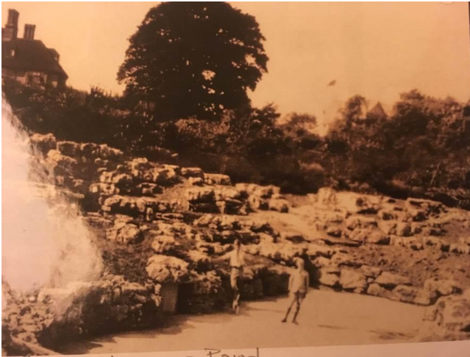
Figure 14. Copy of Terry family photograph during rock garden pool construction, undated. Emailed by Terry family to Goddards, July 2019, after author's request
