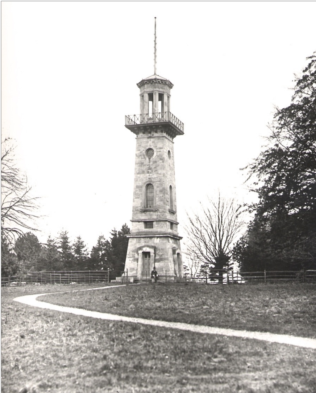
Figure 13 – Grimston Tower in 1872, designed by Decimus Burton c.1840, with gravel path through parkland from the pleasure grounds. Source and copyright © John Fielden Archive
