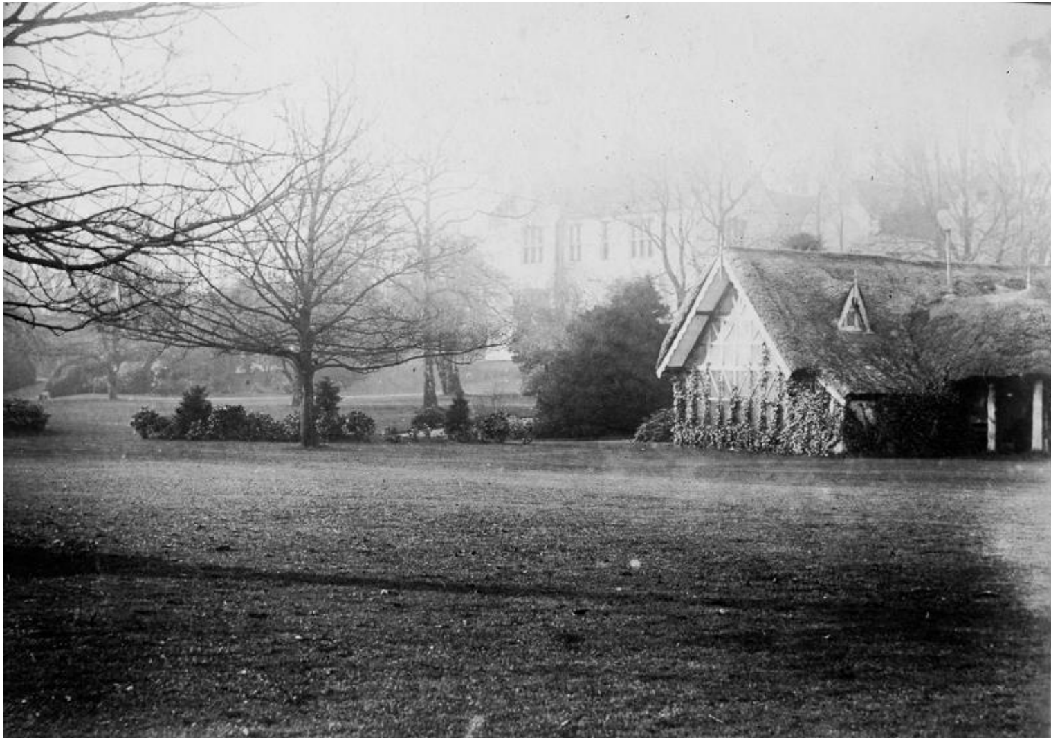
Figure 12 - Thatched Aviary, before reroofing in slate and removal of porch. Reproduced by permission of MFTTA
