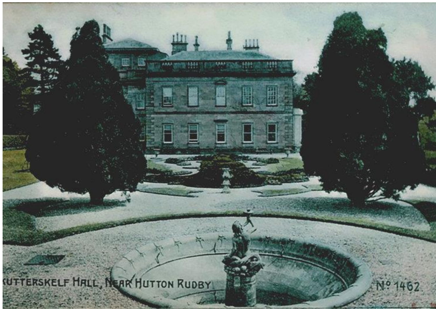
Figure 5 – Skutterskelf Hall terraced garden, early 20th century. Source Rudby Hall.
