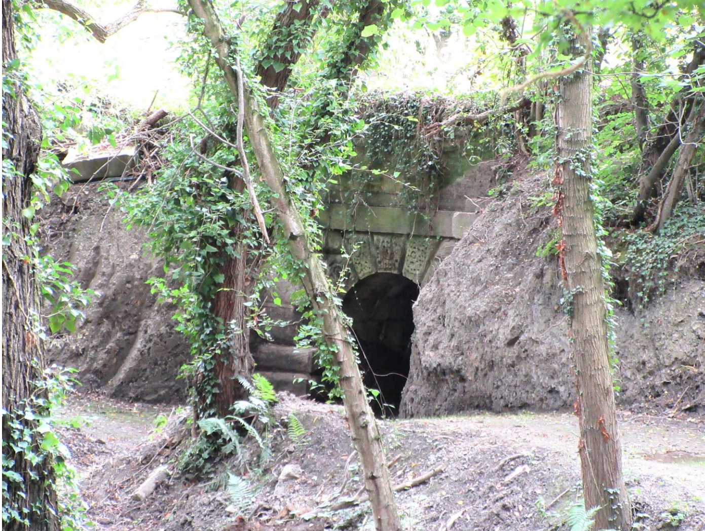
Figure 18. Bridge over Seckar Dike viewed from Mill Lane. Author's photograph, August 2024.
