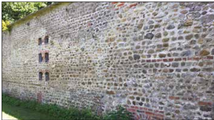
Figure 3: Rear of northeast wall of kitchen garden showing the old flues indicating a heated wall.
