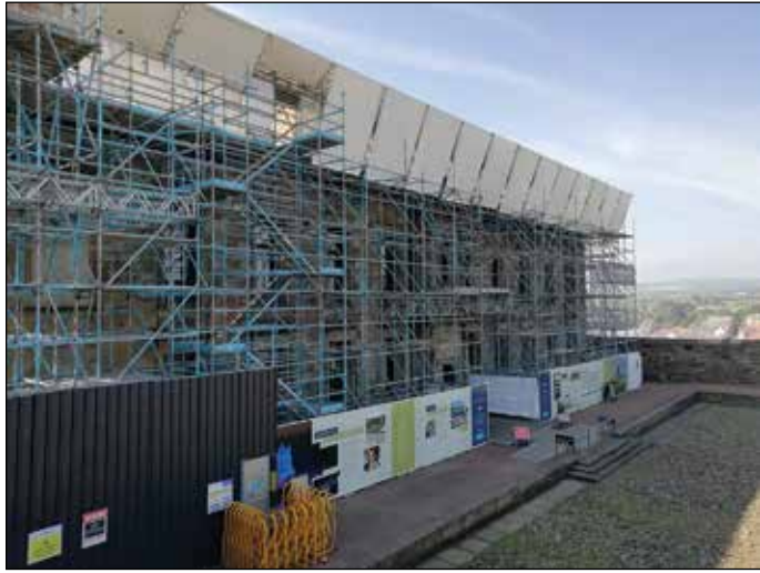
Whitby Abbey Cholmley House/Banqueting House/ Visitor Centre with scaffolding for roof replacement. (Courtesy English Heritage)
