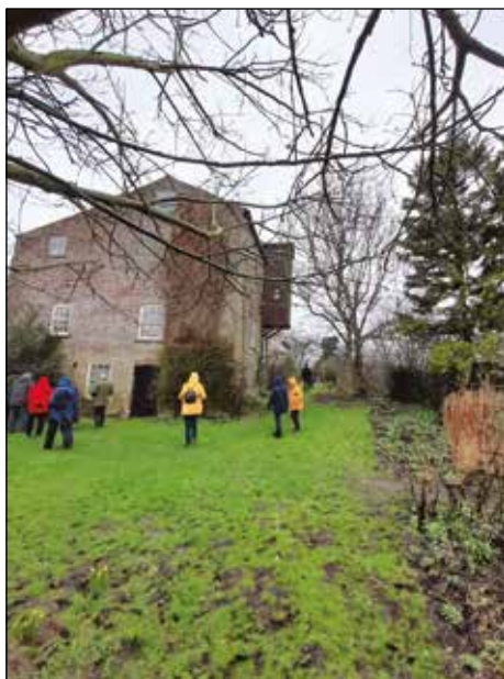
Mill building from the East
