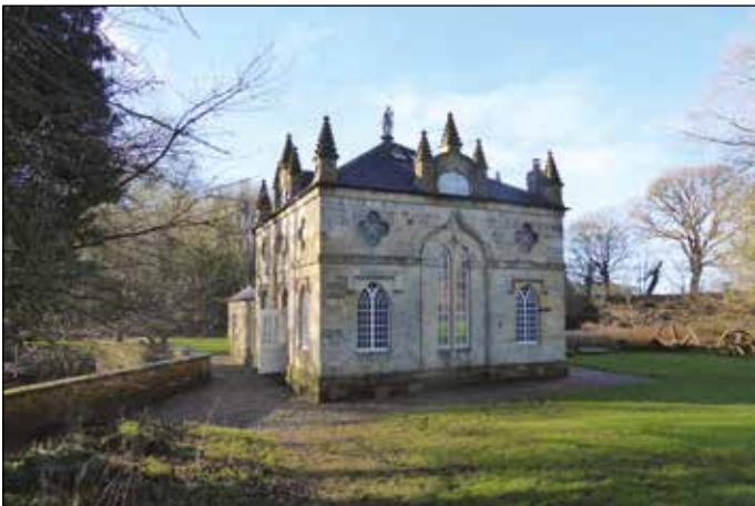
Howsham Mill from east (Photo © Val Hepworth, 2024)
