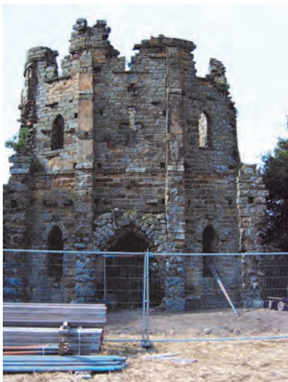
Mowbray Castle Work in Progress
