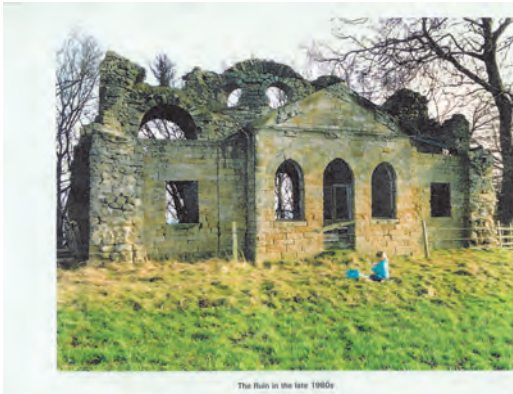
Derelict Banquet House 1980's
