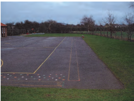
Fig 1 - Before work commenced in grounds of Kirkby & Gt Broughton School
