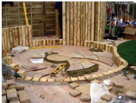
Leeds City College garden at Great Yorkshire Show - mid-build
