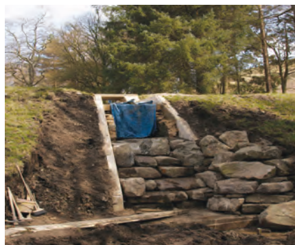
End of Day 4: the original structure is being camouflaged with weatherworn rocks ( Photo: Anne Tupholme )
