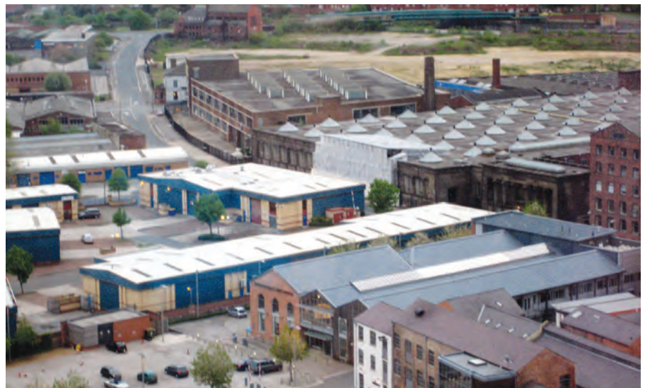
Fig. 3. Marshall’s Mill and roof, with façade under conservation (Photo: Richard Knight)
