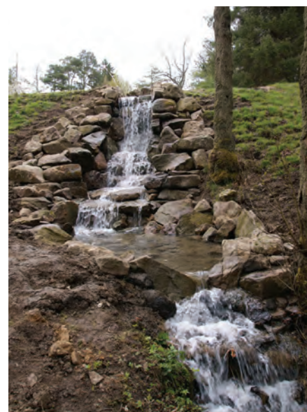
The water falls into a new pool before rejoining Tarn Ghyll Beck ( Photo: Anne Tupholme )
