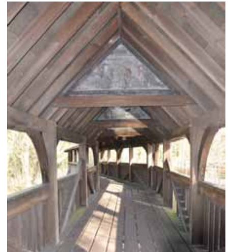
Interior of Lucerne Bridge (photo P Dawson-Brown)
