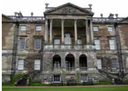
Sandbeck: East front of Paine's mansion (photo D Knight)
