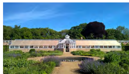
Restored Scampston Conservatory, 2015.
