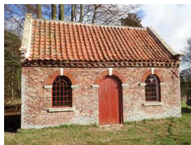
One of the horse shelters at Scampston. (Photograph: Margaret Nieke).
