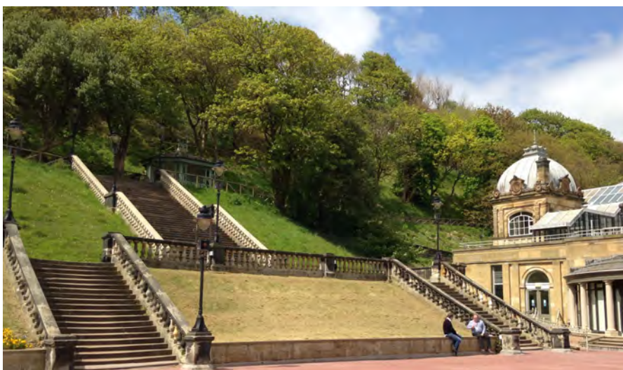
Image: Paxton shelter at top of steps
