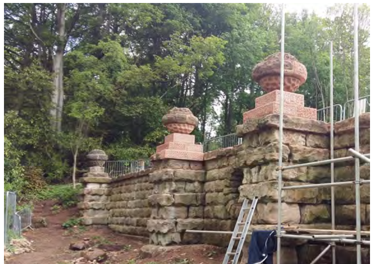
Image: The restoration of the dam.
