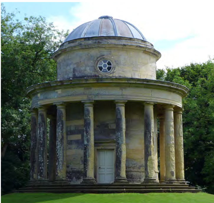
Tuscan Temple, Duncombe Park, before restoration Image: Jake Duncombe
