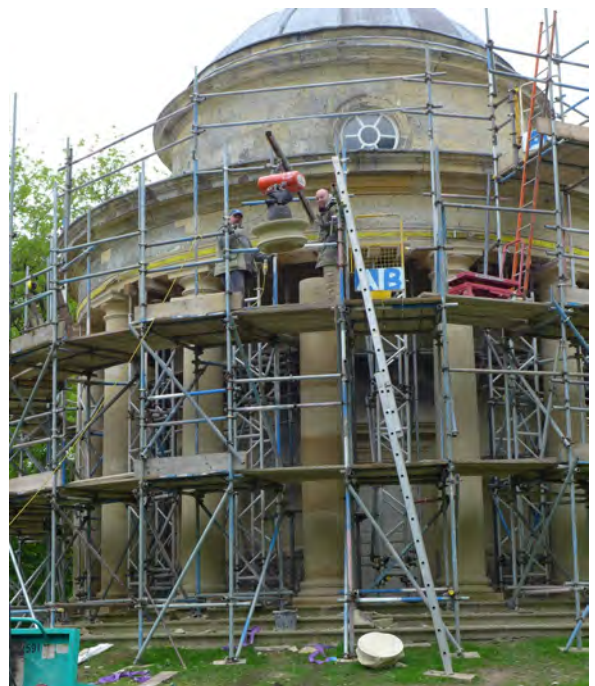
Tuscan Temple, Duncombe Park: the last capital being lifted onto the last column. Image: Jake Duncombe
