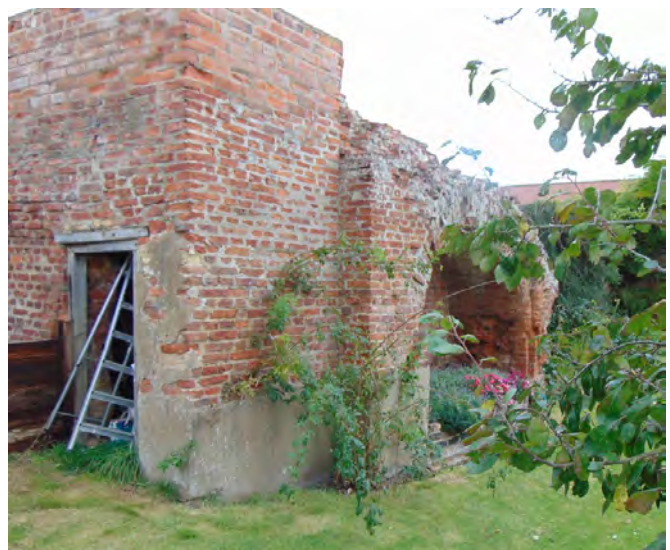
Brick structure across moat - possible viewing tower
