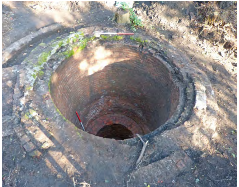
Fully excavated ice well at Carlton Towers, looking south.
