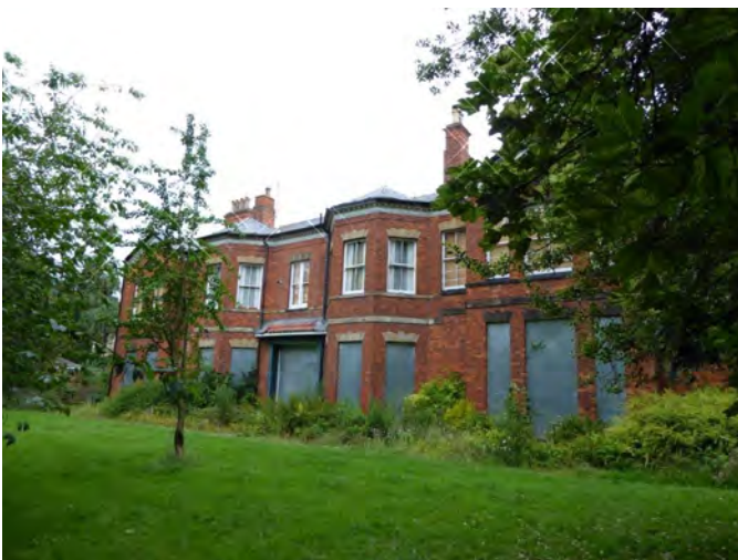
Thwaite Hall: the entrance front from the south/south-east (Image: Val Hepworth)
