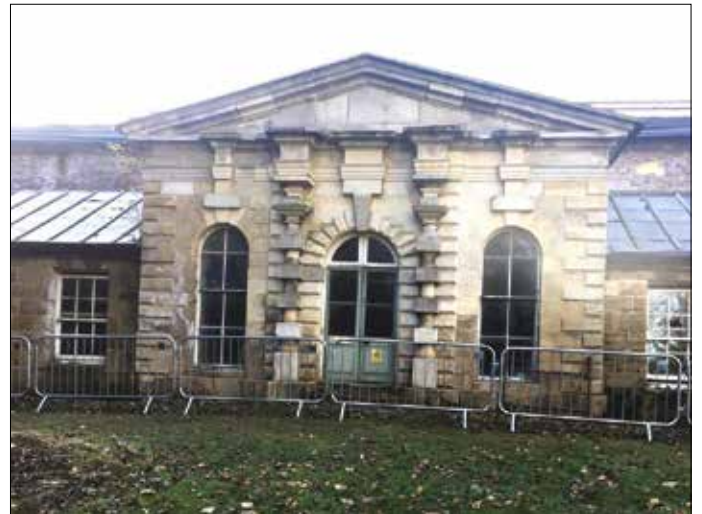
Rear elevation, November 2021: no roof, holes in the wall, unsafe to enter
